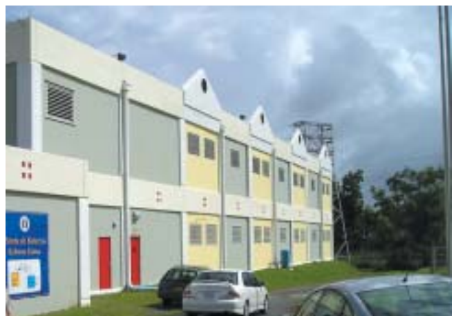
Exhibit 7.3 PREPA's BESS facility, Sabana Llana, PR (source: PREPA)
