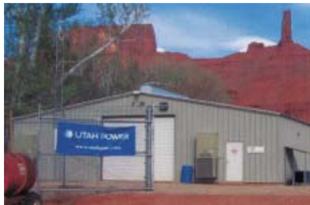
Exhibit 7.15 Vanadium redox flow cell BESS facility at Castle Valley, UT (source: ESA/VRB)
