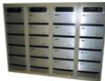
Exhibit 8.2 Cobasys NiGEN rack-mounted ES substation installation
